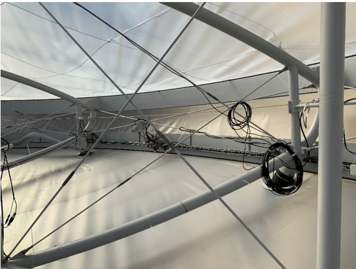
Inside view through the steel structure.
