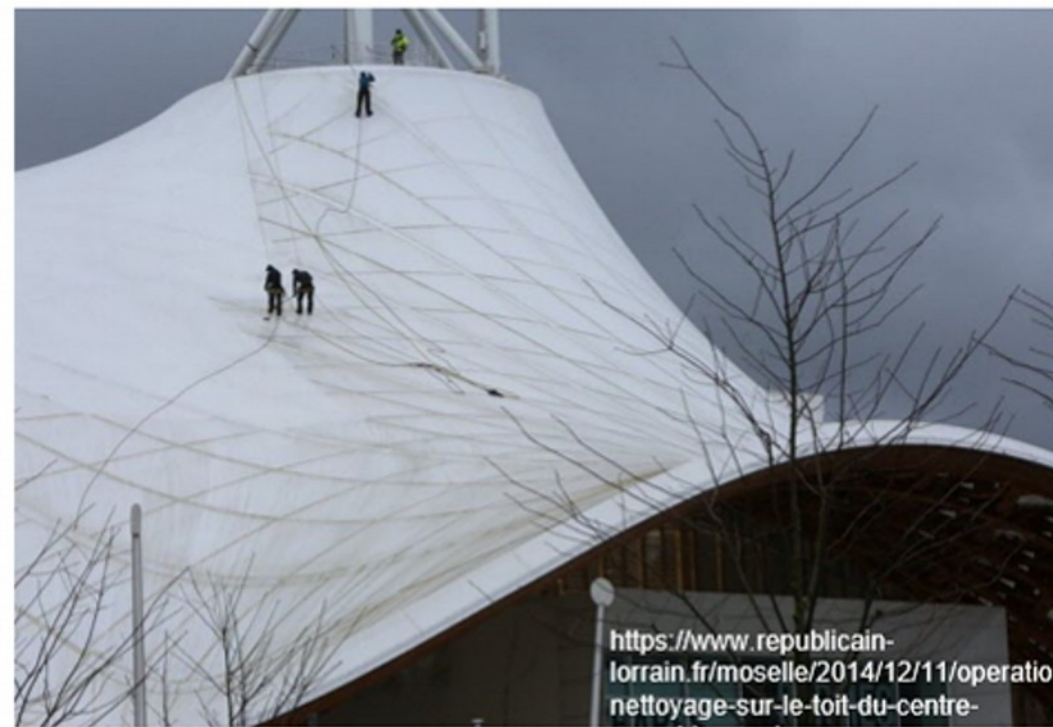
Glass/PTFE project in France
