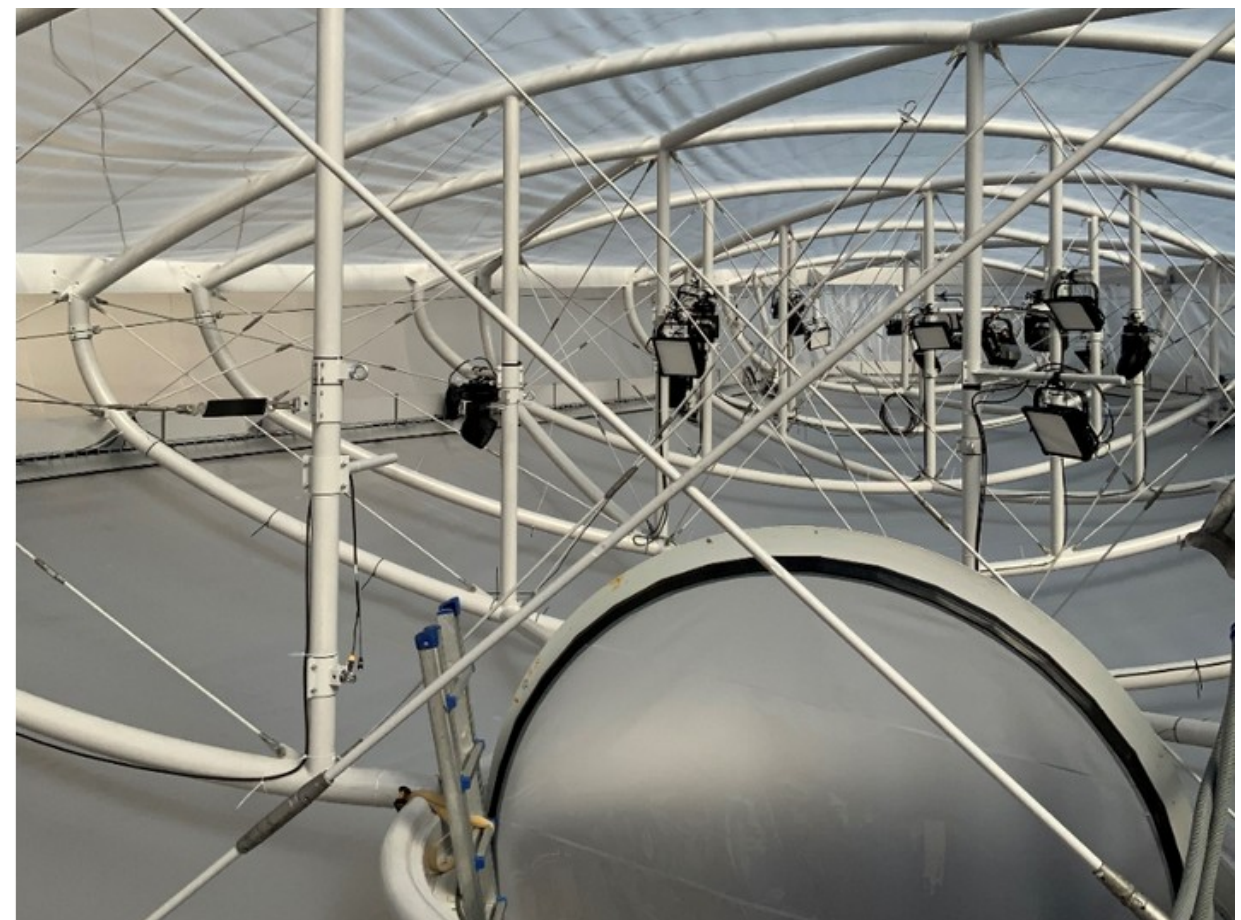
Inside view with the opening for maintenance and light control. (without air pressure)
