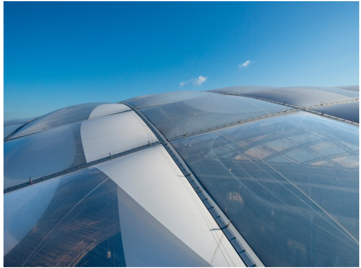
The printing on the cushions ensures that sunlight is reflected, which prevents an excessive heat on the inside.
