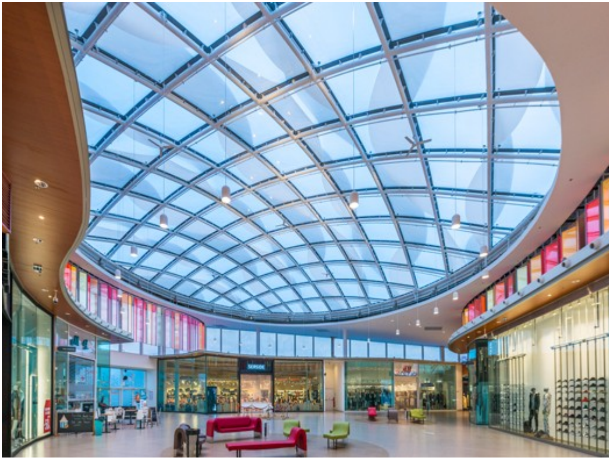
The inner and outer layers of the 3-layered ETFE air-filled cushions are partly printed with organic lines and zones.
